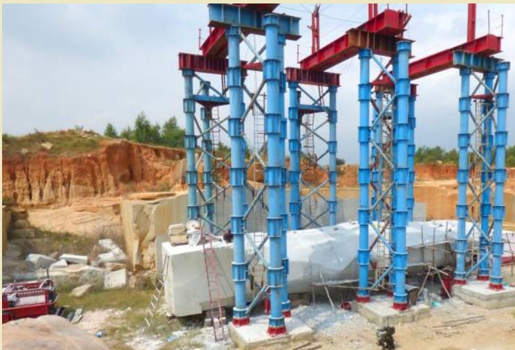
Illustration of tower system used for tilting of semi-carved statue block
